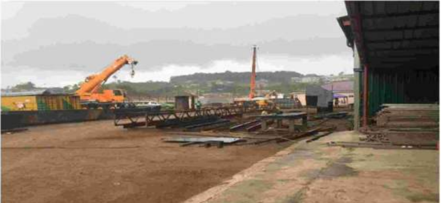
Fabrication of Stacker Conveyors for ArcelorMittal
