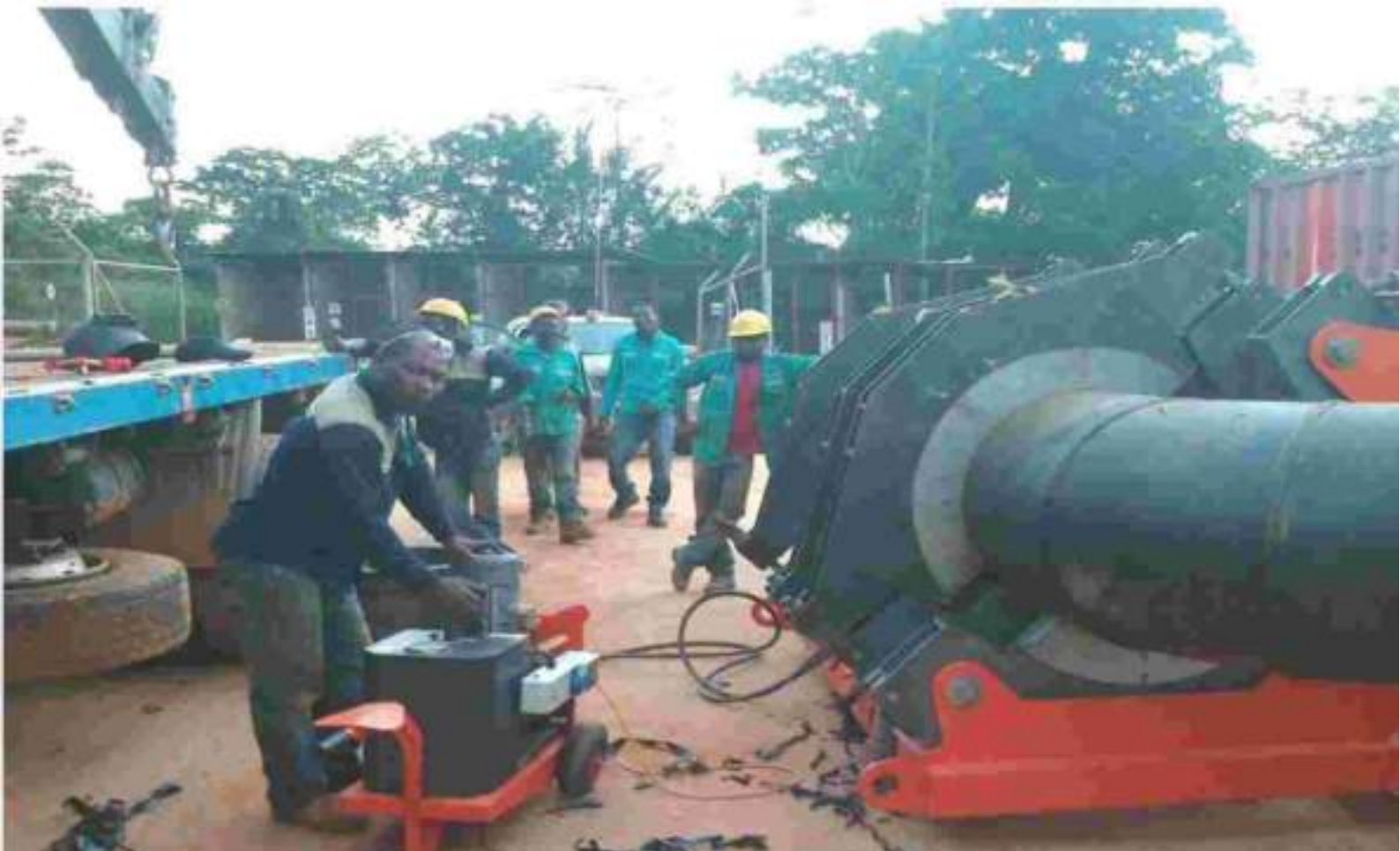
USION OF 800mm HDPE PIPES FOR NEWMONT GOLD CORP AKYEM MINES
