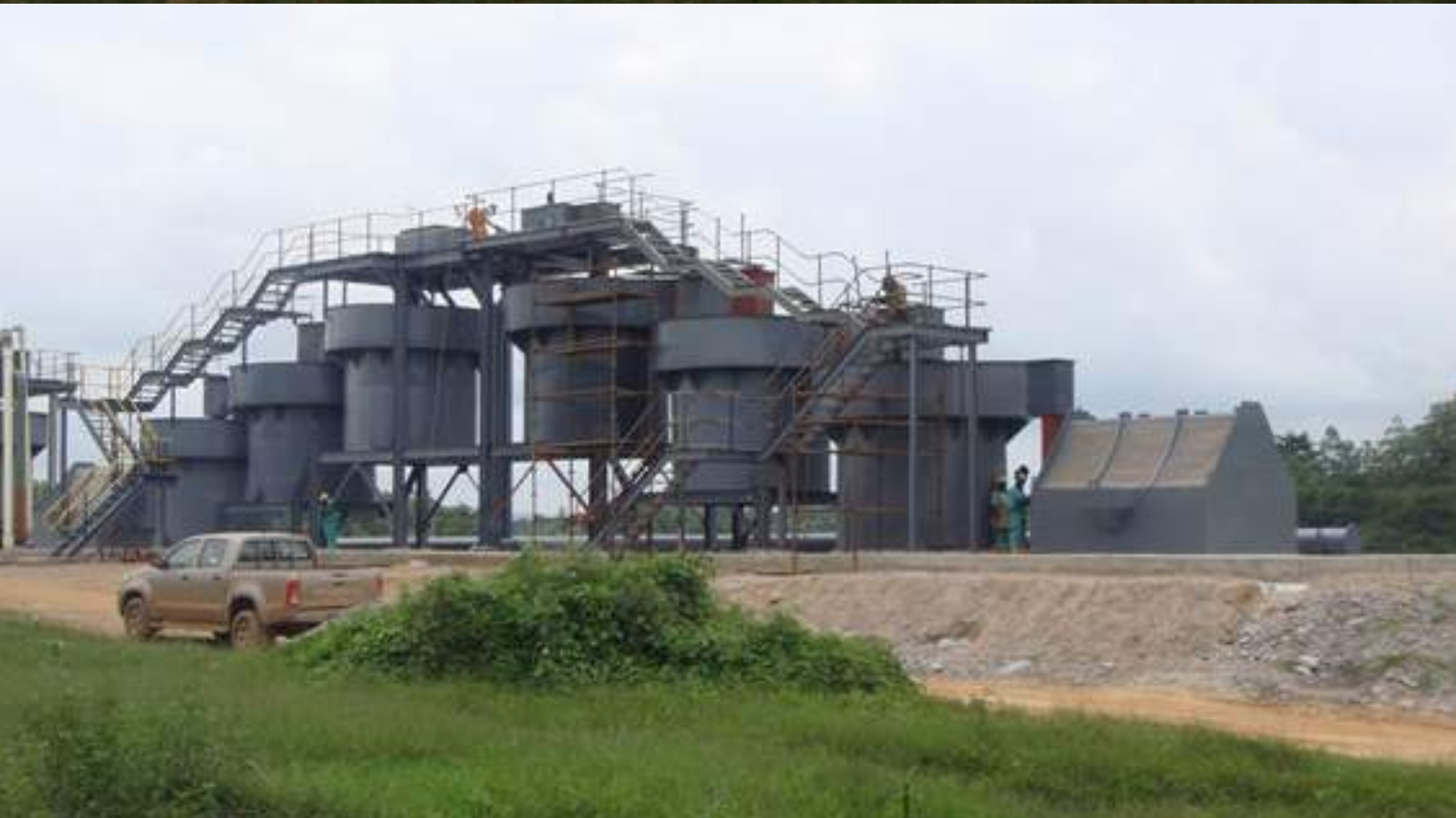
COMPLETE SET OF CASCADE COLUMNS AND SCREENS FOR GOLDFIELDS GHANA
