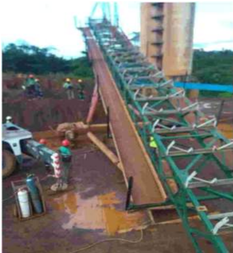
Installation of Stacker Conveyor and chutes for Arcelor Mittal
